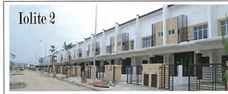
Iolite 2 Double Storey Terrace (20' x 70') 2,027 sq.ft. | Work In Progress (%) 94%
