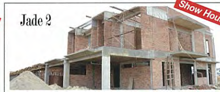
Jade 2 Double Storey Terrace (22' x 75') 2,227 sq.ft. | Work In Progress (%) 41%
