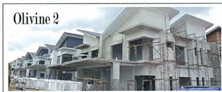
Olivine 2 Double Storey Cluster 2 (32' x 75') 2,764 sq.ft. | Work In Progress (%) 57%
