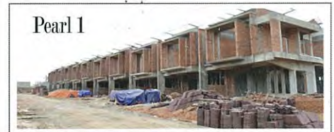
Pearl 1 Double Storey Terrace (26' x 80') 2,588 sq.ft. | Work In Progress (%) 37%
