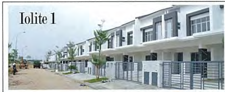
Iolite 1 Double Storey Terrace (20' x 70') 1,949 sq.ft. | Work In Progress (%) 98%
