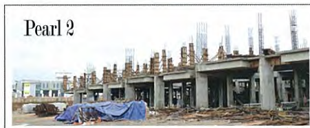
Pearl 2 Double Storey Terrace (24' x 80') 2,473 sq.ft. | Work In Progress (%) 24%
