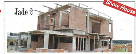
Jade 2 (Type B) Double Storey Terrace (24' x 75') 2,507 sq.ft. | Work In Progress (%) 41%
