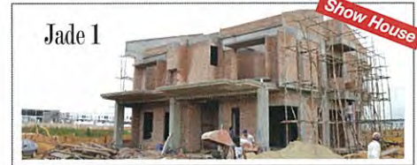
Jade 1 Double Storey Terrace (22' x 75') 2,209 sq.ft. | Work In Progress (%) 37%
