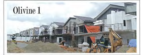
Olivine 1 Double Storey Cluster 1 (35' x 75') 2,669 sq.ft. | Work In Progress (%) 57%
