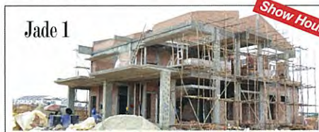
Jade 1 (Type B) Double Storey Terrace (24' x 75') 2,552 sq.ft. | Work In Progress (%) 37%
